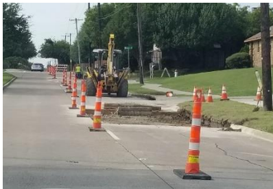
Construction Companies Group (CCG) is currently working on panel replacements on Rowlett Rd. between Miller Road and Dogwood Trail.
